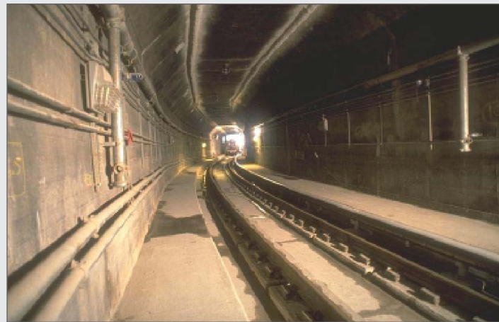
Figure 4-5 Empire Tunnel (Amtrak)
