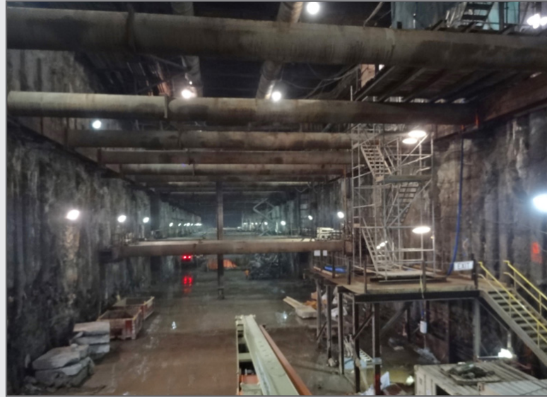
Figure 4-26 Cut-and-Cover Strutted Excavation, Second Avenue Subway Project
