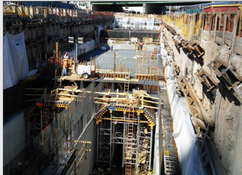
Figure 4-28 Hudson Yards Concrete Casing Project
