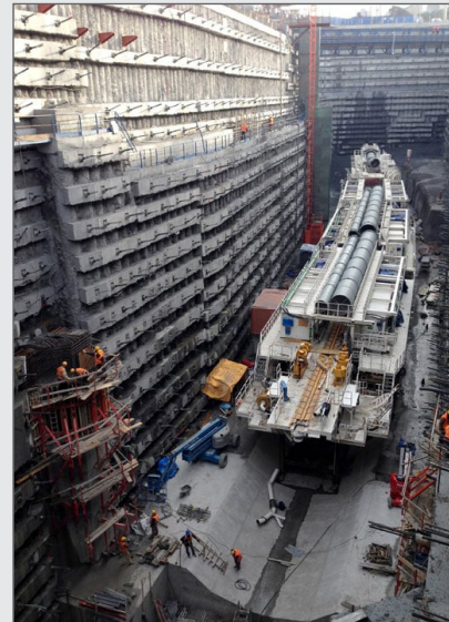
Figure 4-29 Cut-and-Cover Portion of Eurasia Tunnel, Istanbul, Turkey
