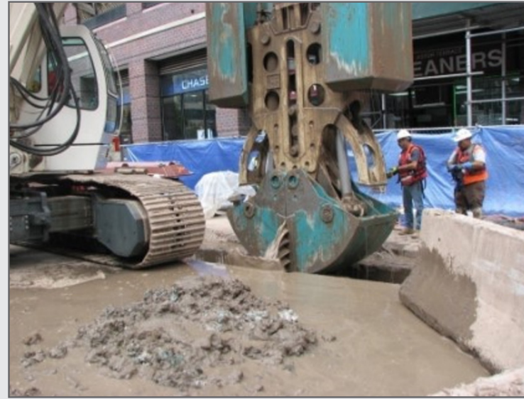
Figure 4-27 Slurry Wall Construction Second Avenue Project
